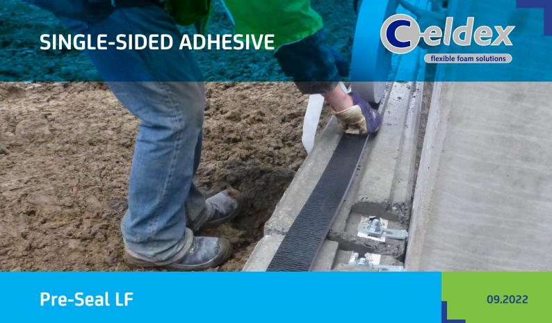
Celdex Pre-Seal LF is a semi-closed cell polyurethane foam tape with excellent airtight and insulating properties. The product is suitable as an airtight sealing and thermal insulation for irregular surfaces. Pre-Seal LF is airtight, in conformity with NEN 3660/3661 and is highly versatile in varying joint connections.
